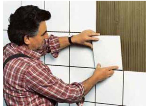
Reliable laying of tiles in the thin-bed method with MasterTile 15
